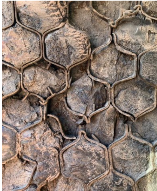
Inherent in its design, closed cell systems allow for pathways that reach behind the lining.
