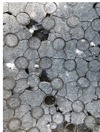
Refractory with missing chunks.
