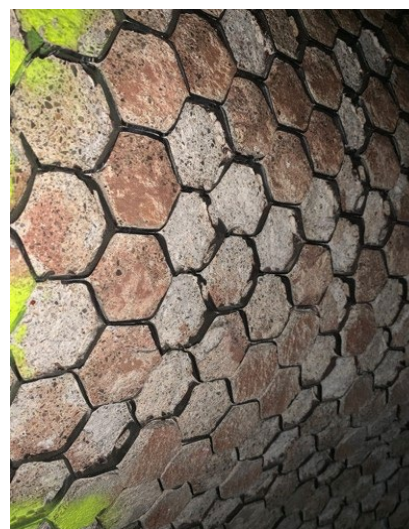
Refractory spalling, called biscuiting.
