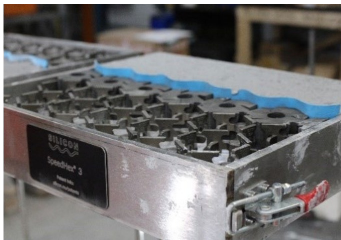
Semi-closed cell system refractory installation with an intentional cold joint.
